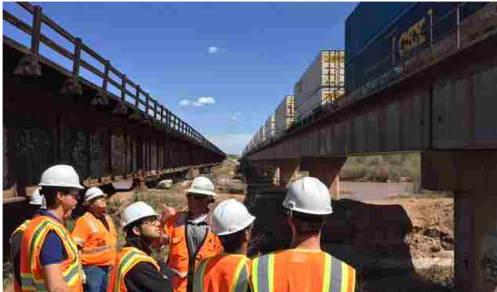
Fig. 1.3. Railroad bridge visual inspection.
