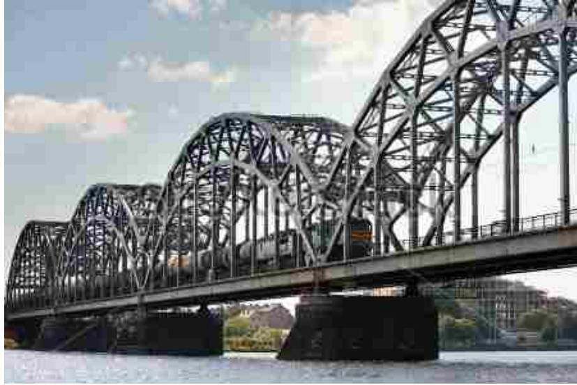
Fig. 1.4. Railroad bridge under service load.
